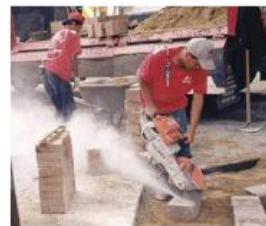
Dry sawing concrete
